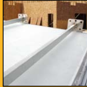
Roof Mounted Ladder Racks
